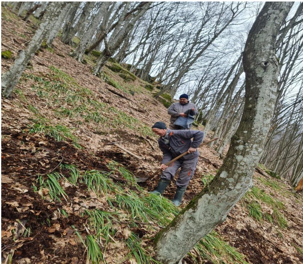
Figure 5: Trench excavation is carried out manually because the terrain is too steep to apply an excavator.
